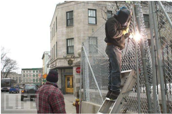
Quebec City 2001, Building the Security fence
